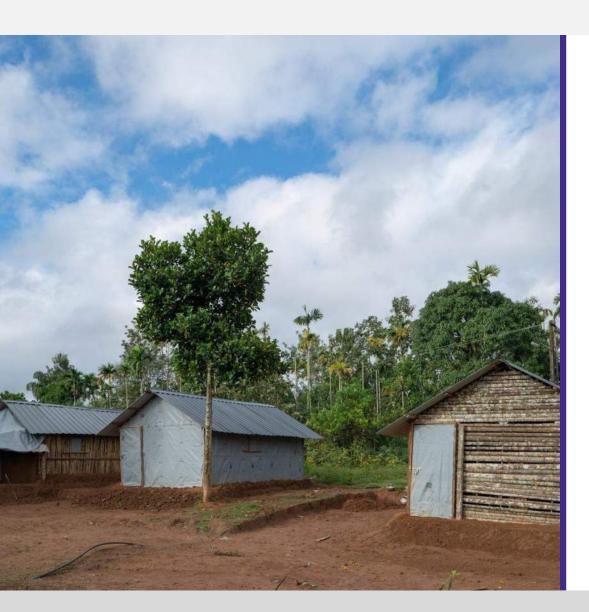
The *Structure* approach offers **low-cost**, transitional tentage for forcibly displaced people, capable of lasting the **duration of displacement** through upgrading with local materials. Its modular metal framework can be deployed with a tarpaulin cover and serve as an **emergency shelter** in the immediate aftermath of a disaster or conflict.
