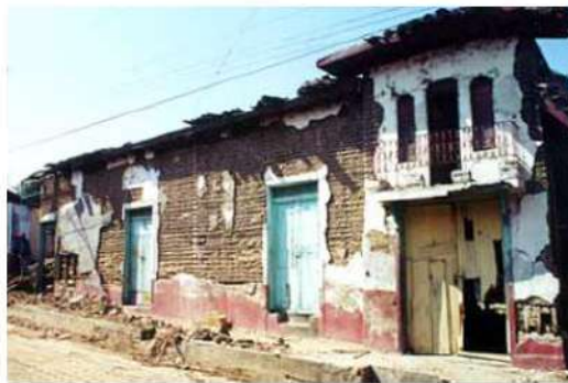
Figure 9. Damage to bahareque in San Vicente caused by the 13 February 2001 earthquake
