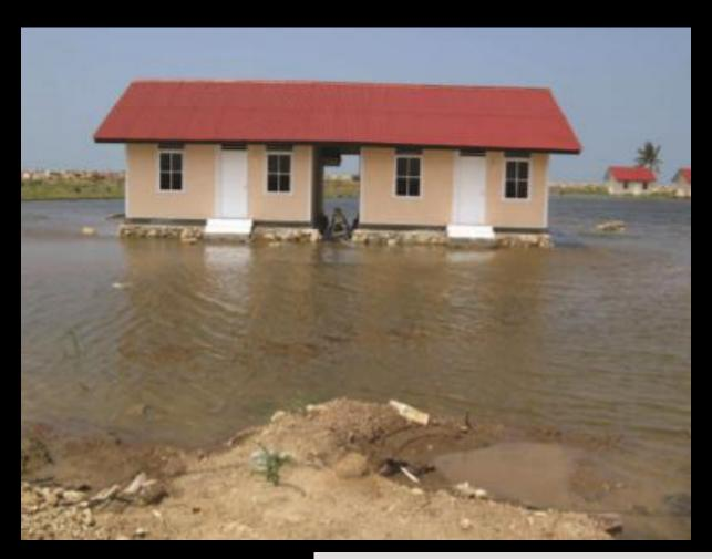
Shelter construction. The rush to construct houses after the tsunami resulted in some new homes being constructed in unsafe areas as shown in in this photo.. Flooded homes can lead to increased risk of water-bourne disease and unsafe living conditions. Note: a newly constructed sea wall in the background aggravates the problem because it prevents rainwater from flowing out to sea. (See Module 4, Green Guide to Strategic Site Selection and Development for ways to address this issue)
