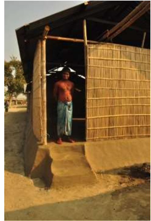
Figure 2: Houses built on raised plinths in Morigaon
